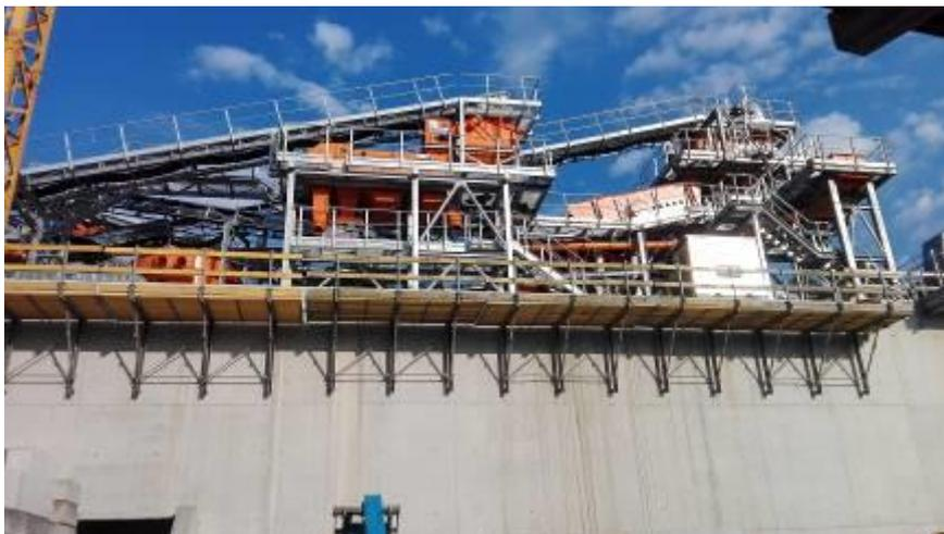
*Bild 2: The silos were integrated in the concrete construction and the processing unit was placed above in the steel construction (picture taken shortly before establishing the housing).*
